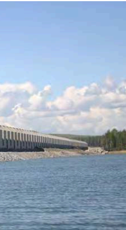
The Vuosaari Harbour project in Finland, to be completed in 2008, is one of Europe's largest harbour projects with 3.4km of new quay wall. Rudus delivered the concrete used in the construction of 675 high-quality quay elements at the site.
