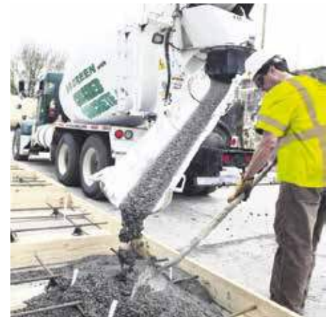
Harrison Construction, which has operations in Tennessee and North Carolina, US, has invested in an award-winning mobile crushing operation to recycle and reuse materials that would otherwise be discarded, increasing the sustainability of its products and business.
